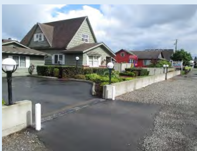
Local Flood Wall
