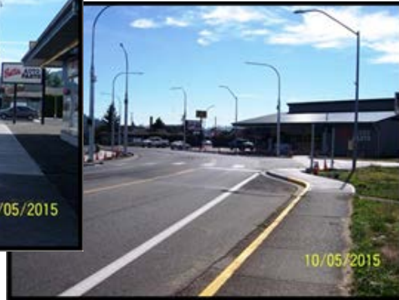
Above and right, Main & Yew Traffic Signal
