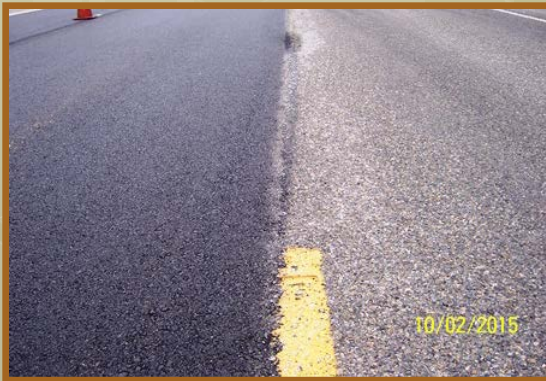
Left—new asphalt on Galvin Rd. Right —chip seal done by City summer of 2014
