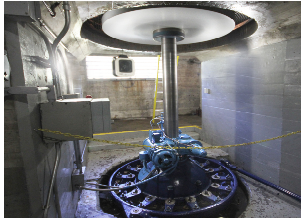
Hydro-turbine governor and shaft
