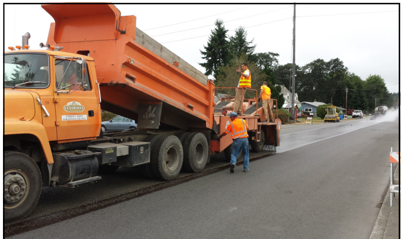
Chip sealing protects road surfaces, furthers road life expectancy.
