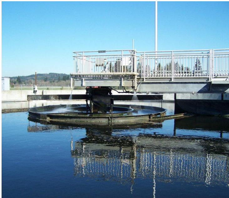
Sewer treatment plant clarifier
