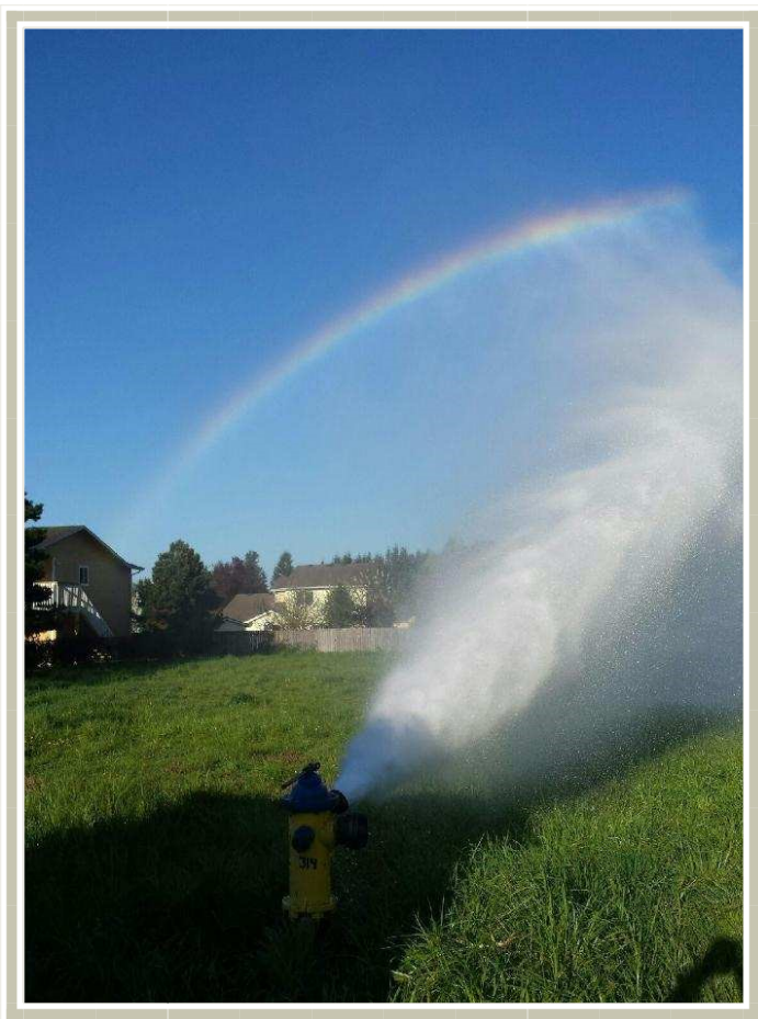
Flushing Hydrants
