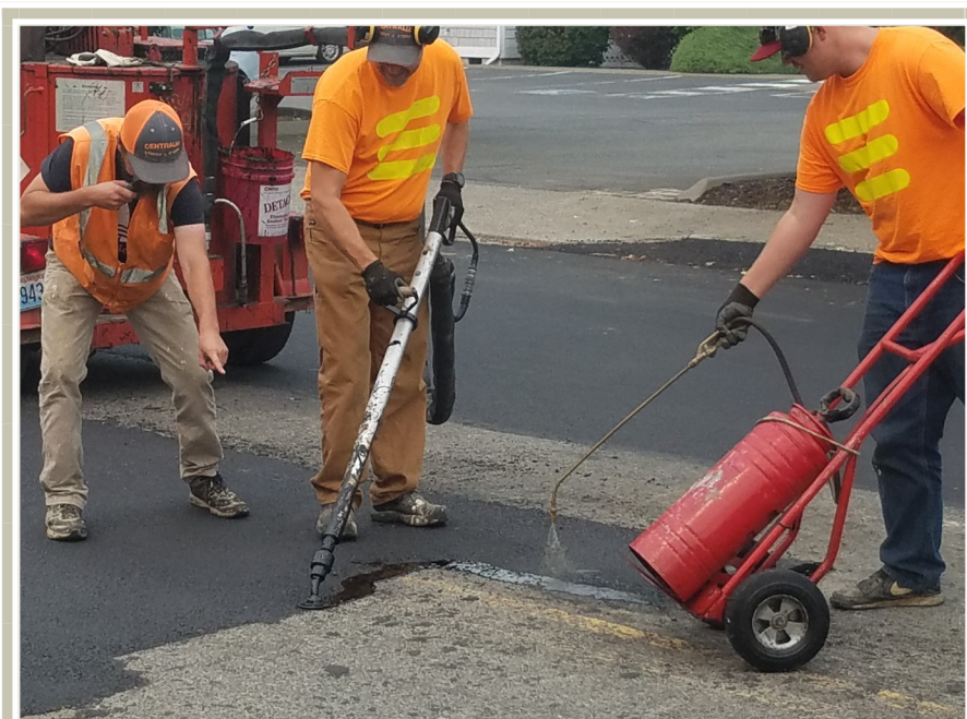
Street Crew working on Asphalt patches
