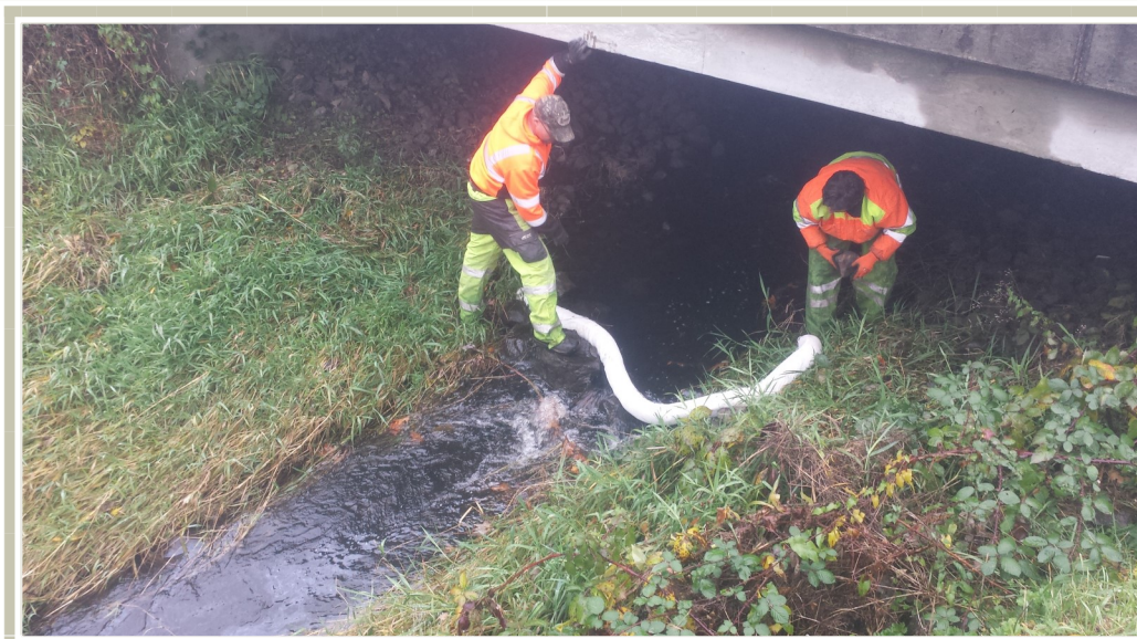
Oil boom being placed in China Creek to collect oil from the surface.
