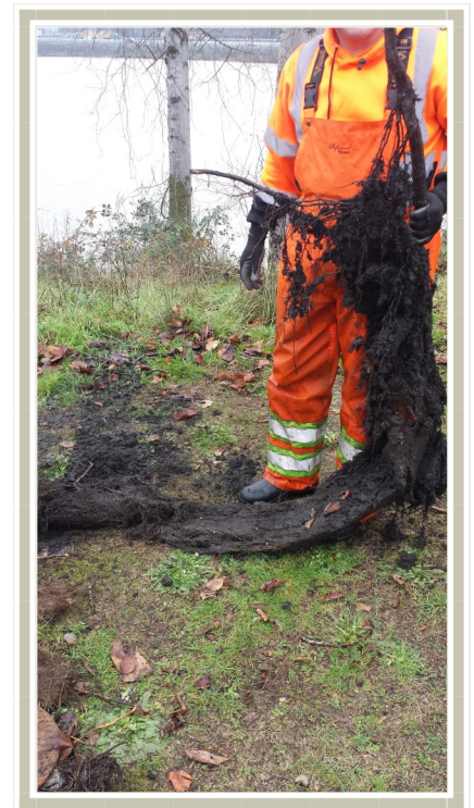
Tree roots removed from storm sewer line.
