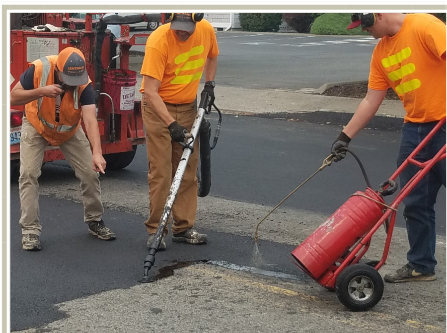
Street Crew working on Asphalt patches
