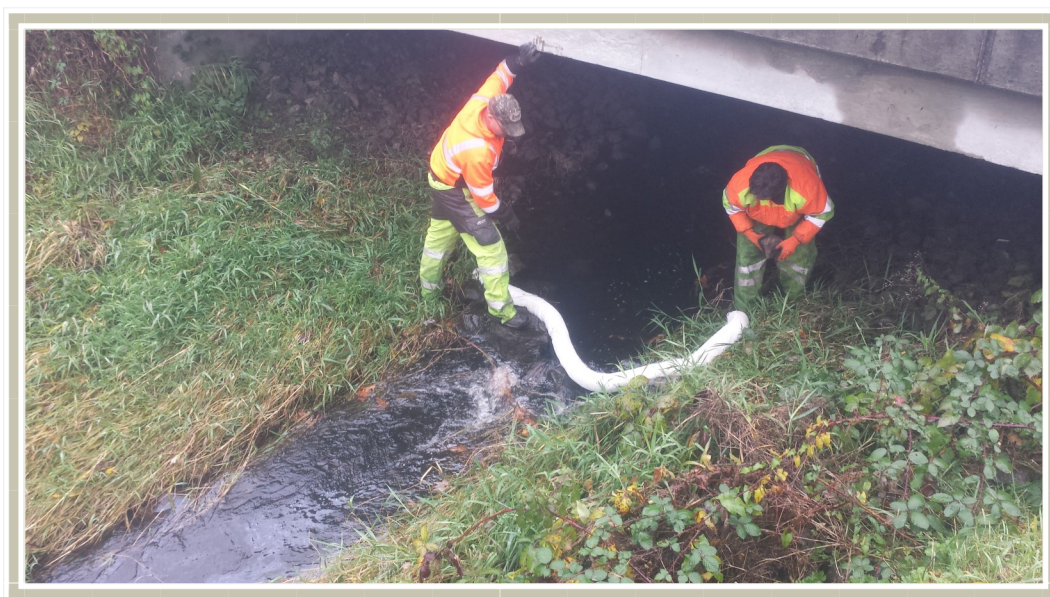
Oil boom being placed in China Creek to collect oil from the surface.
