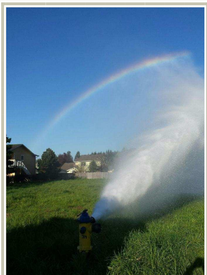
Flushing Hydrants
