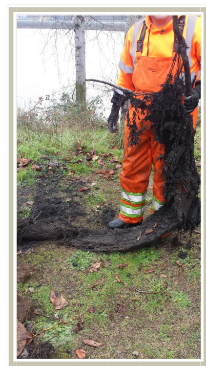
Tree roots removed from storm sewer line.
