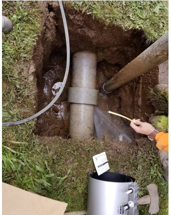
10 inch water main leak at N. Washington and 4th
