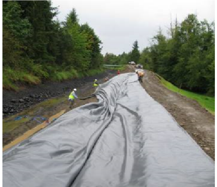
Installing liner along canal embankment
