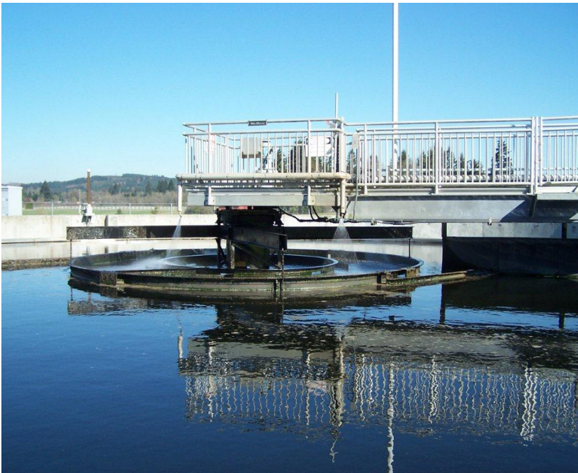
Sewer treatment plant clarifier
