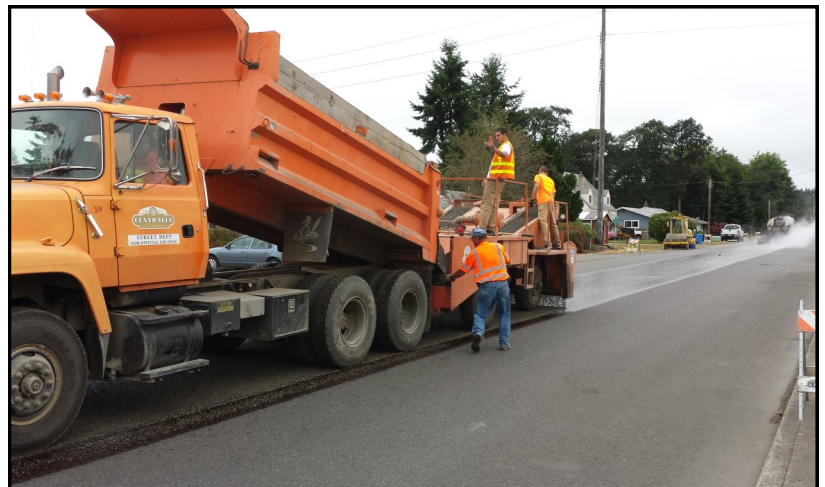
Chip sealing protects road surfaces, furthers road life expectancy.
