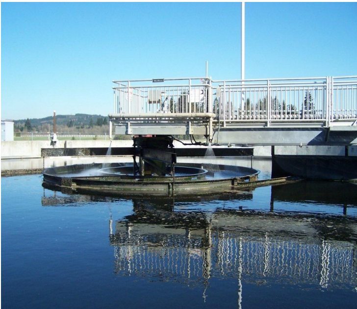
Sewer treatment plant clarifier
