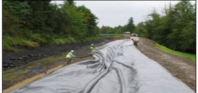
Installing liner along canal embankment
