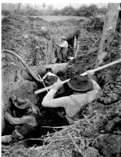
Figures 6 and 7: Workers digging trench for laying the pipe
