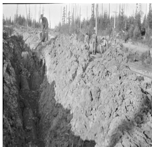
Figures 6 and 7: Workers digging trench for laying the pipe
