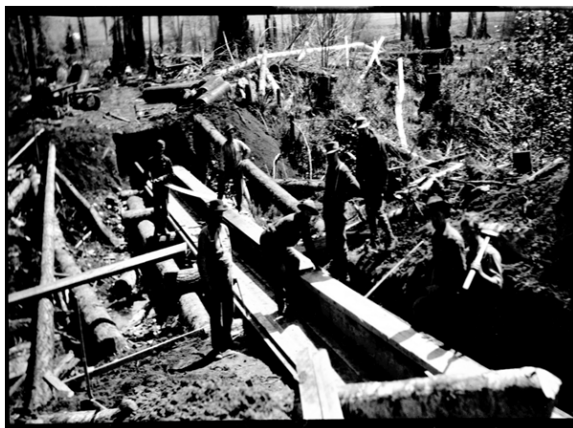
Figure 8: Workers laying 14-mile pipeline from the Newaukum River. Figure 9: 14-mile pipeline
