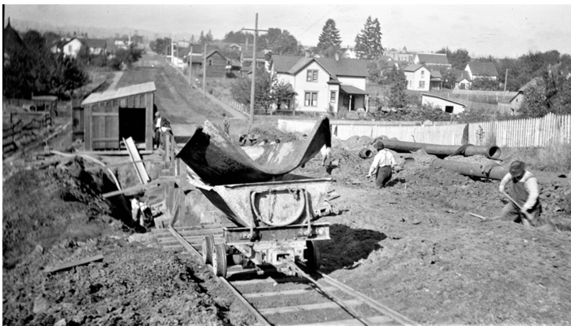
Figure 2: Locust Street torn up to transport equipment to the site and workers digging trenches for pipe.
