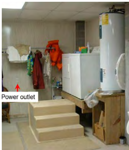
The washer, dryer, and water heater were elevated in this wet floodproofed garage.
