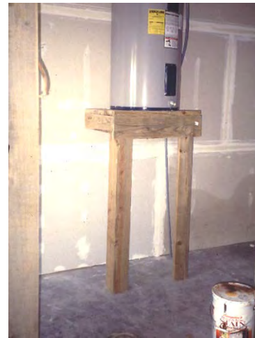
The owner replaced a flood damaged water heater with a shorter one and elevated it.
