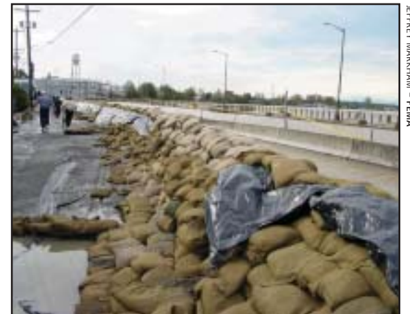
Sandbag wall in Mount Vernon, Washington
