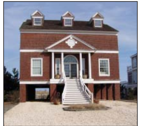
Coastal home elevated to avoid future flooding.
