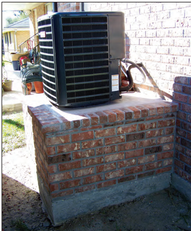
Figure 3-1. Air conditioning compressor elevated on a pedestal.
