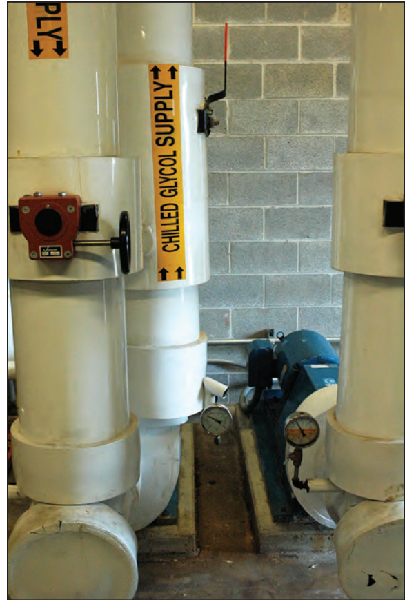
Figure 5-4. Chilled water pump, Georgetown, Delaware.
