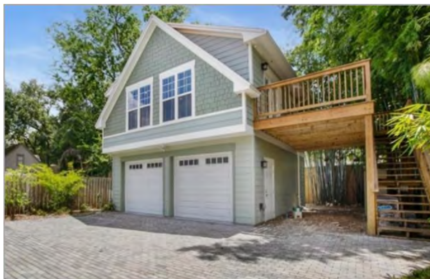
Figure 16: Elevated Accessory Residential Structure, with Enclosure
