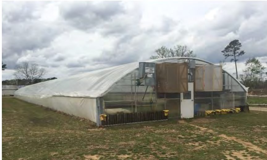
Figure 13: Greenhouse with Flexible Sides and Removable “Roof”
