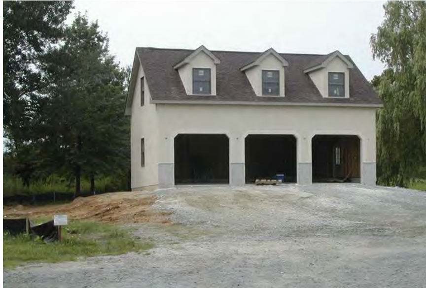
Figure 21: Three-Car Garage Elevated on Fill
