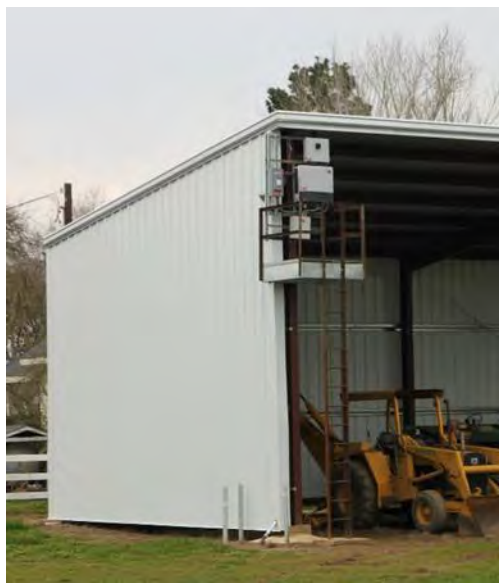
Figure 24: Elevated Electric Service and Equipment
