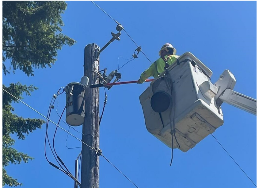
Installation of Wildlife Resistant—Transformer Insulator
