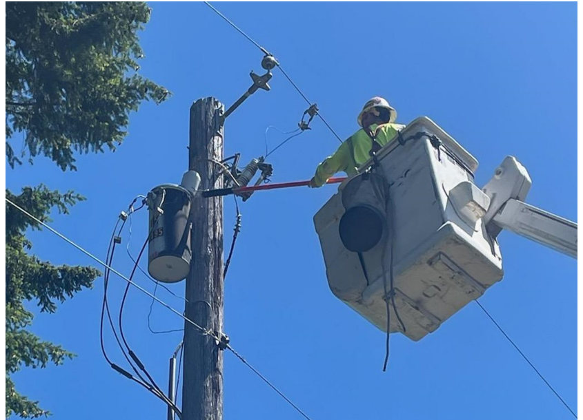
Installation of Wildlife Resistant—Transformer Insulator
