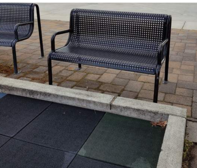
The curb at the accessible surfacing creates a barrier and trip hazard
