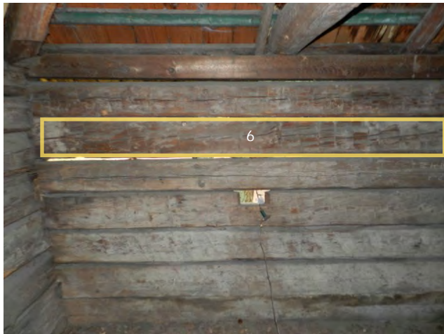
Interior of log 6 Hollow in center
