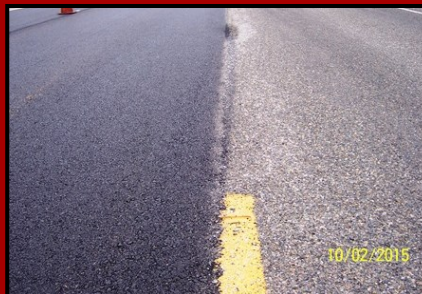
Left side—new asphalt on Galvin Rd.
